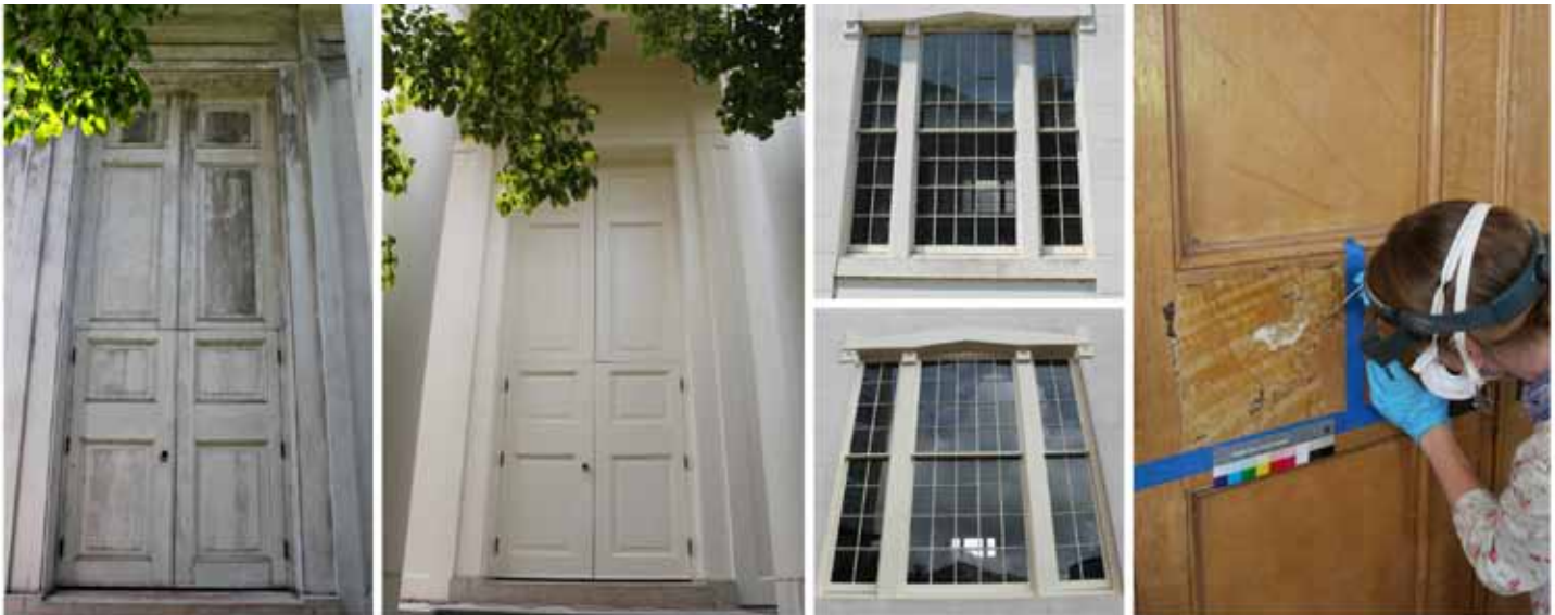
Before and after photos of east portico door and window
